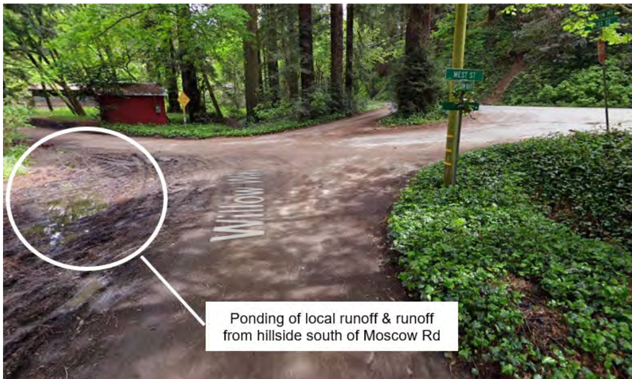
Figure 5-6: Low Point at Willow Road where Runoff from Moscow Road Accumulates
