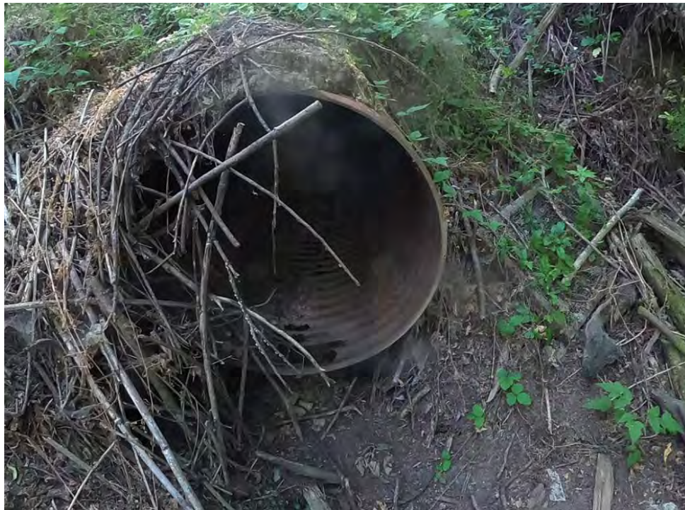
Figure 5-10: Southern Pipe System Outfall (From 6 th Street).
