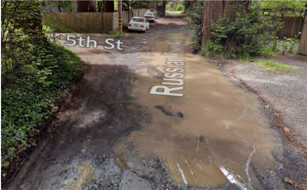
Figure 5-3: Ponded Water at Russian River Ave & 5 th Street
