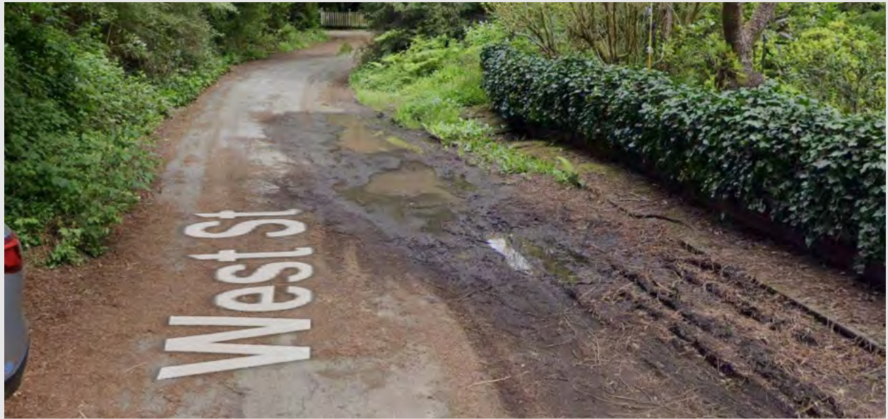
Figure 5-5: Ponded Water and Sediment Buildup on West Street (Between Post Office and East St)
