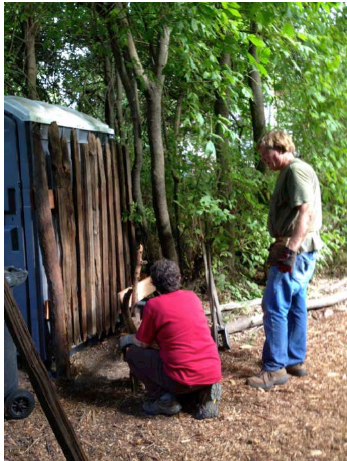
Natalie Robb-Wilder and Rich Holmer work on screening panels.
